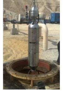
SCHNEIDER WATER SERVICES HAS TOOLING CAPABLE OF DEVELOPING AND REHABILITATING WELLS UP TO 24 INCH DIAMETER.
